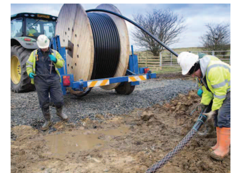
7. Pull cables into ducts
